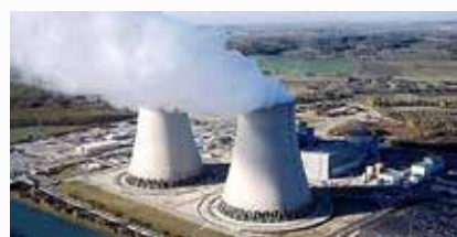
EDF nuclear power station
